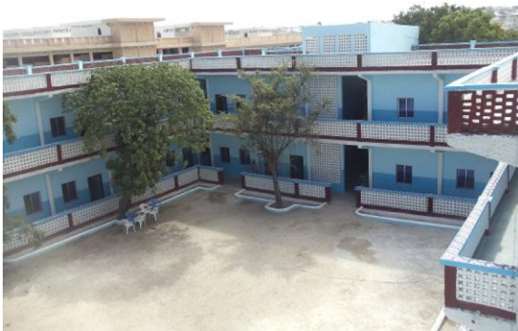
Moalim Jama Secondary School after rehabilitation
