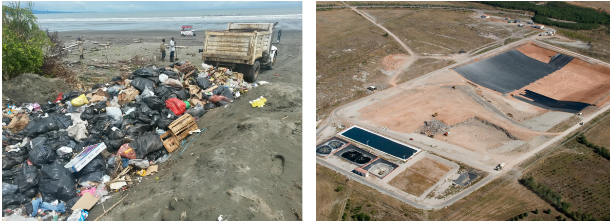
Typical dumpsite in Aruba (left), and new engineered landfill site in West Macedonia, Greece (right). Source: Mott MacDonald
