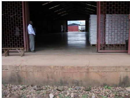
Photo no. 2: ACDI/VOCA Warehouse with Open Doors (This will let birds, rodents, and insects easily gain access into the warehouse)
