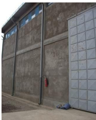
Photo no. 3: Save the Children Warehouse in Adama, Ethiopia showing gaps underneath the door
