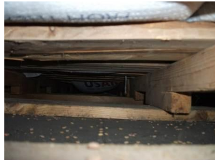
Photo no. 18: Spillage underneath Pallets at a Warehouse in the Free Zone (Djibouti)
