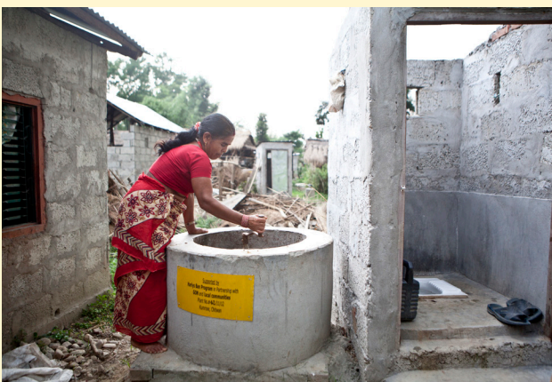
A beneficiary in Kumroj demonstrates how the mixture is churned in the biogas pit, typically constructed next to a toilet.
