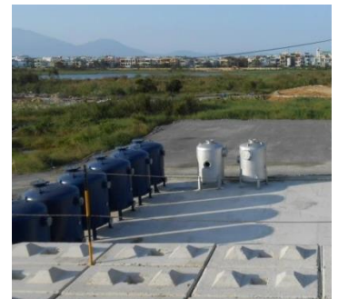
GAC vessels delivered to site (Photo: CDM Smith)
