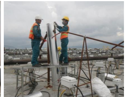
Final construction on top of the treatment structure (Photo: CDM Smith)
