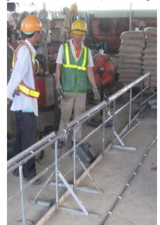
Heater repairs (Photo: TerraTherm)
