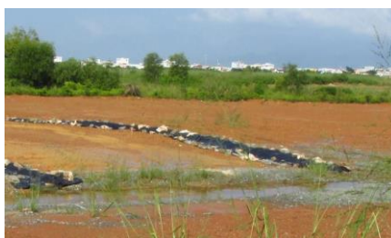
Erosion control measures (Photo: Tetra Tech)
