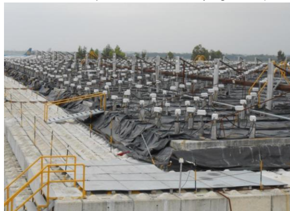
HDPE liner on top of concrete cap
