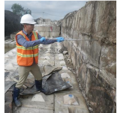
Collecting sample from wall of treatment pile structure. (Photo: CDM Smith)
