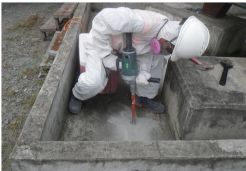
Drilling to collect samples from a concrete pad. (Photo: CDM Smith)
