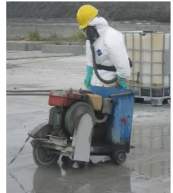
Cutting the concrete pad for disposal. (Photo: CDM Smith)
