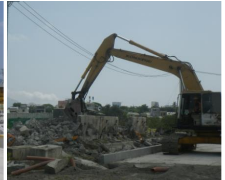
Demolishing structures/elements of the treatment system. left photo: concrete pad of the liquid vapor treatment plant; right photo: cooling tower basin. (Photos: CDM Smith)
