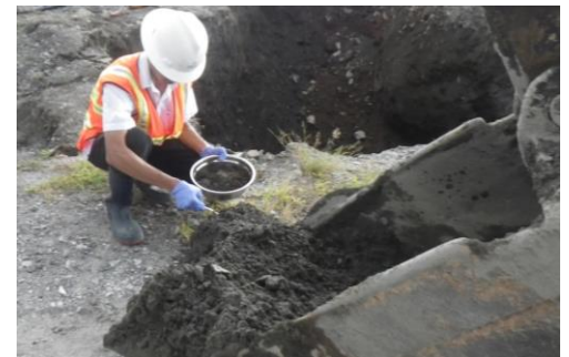
Collecting soil samples to confirm soil beneath the treatment system is clean. (Photo: CDM Smith)
