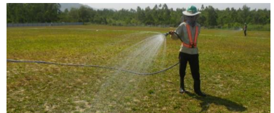
Watering newly planted grass. (Photo: CDM Smith)
