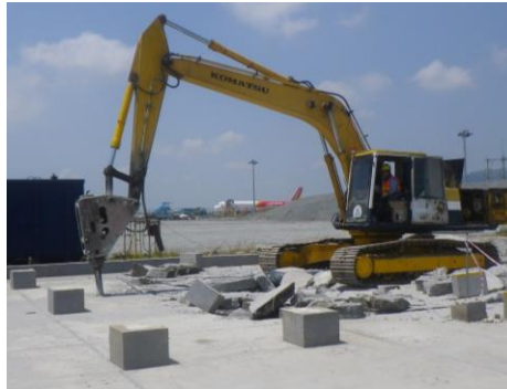
Demolishing structures/elements of the treatment system. left photo: concrete pad of the liquid vapor treatment plant; right photo: cooling tower basin. (Photos: CDM Smith)
