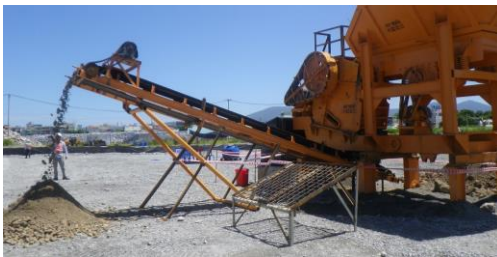
Processing concrete using a crusher (Photo: CDM Smith)
