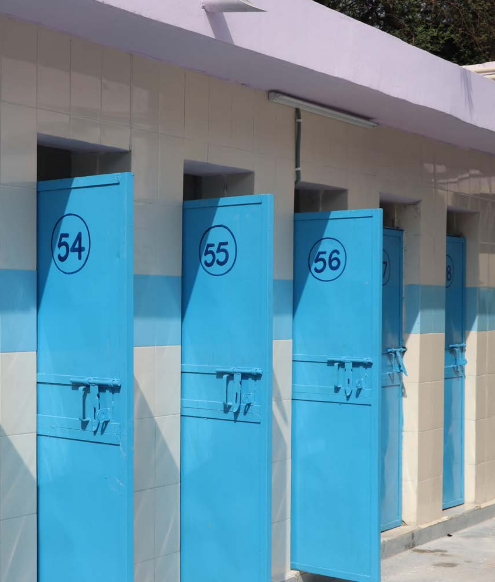
In India as well as in other Asian countries such as Indonesia and Nepal, USAID is supporting efforts to provide community WASH solutions such as these public latrines, when household sanitation is not always feasible or sufficient. In FY 2016 USAID provided 273 basic sanitation facilities in institutional settings. Photo credit: USAID/India
