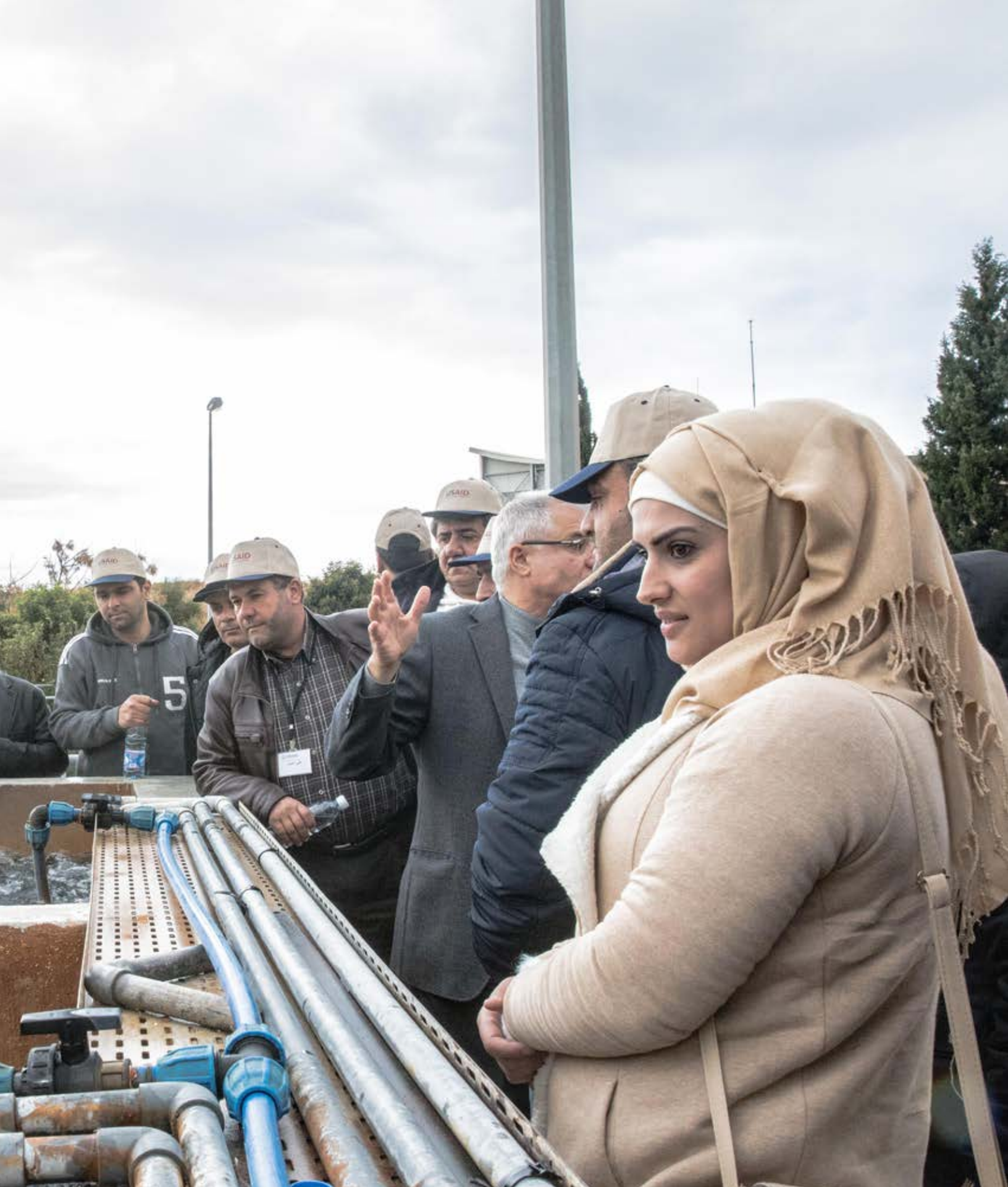
Water operators from the Beqaa Water Establishment tour a water treatment plant as part of a training offered by the USAID-funded Lebanon Water Project on water treatment, including disinfection and lab testing. The 10-day training falls within USAID's main goals of ensuring clean, reliable, and sustainable sources of drinking water. Photo credit: USAID Lebanon Water Project
