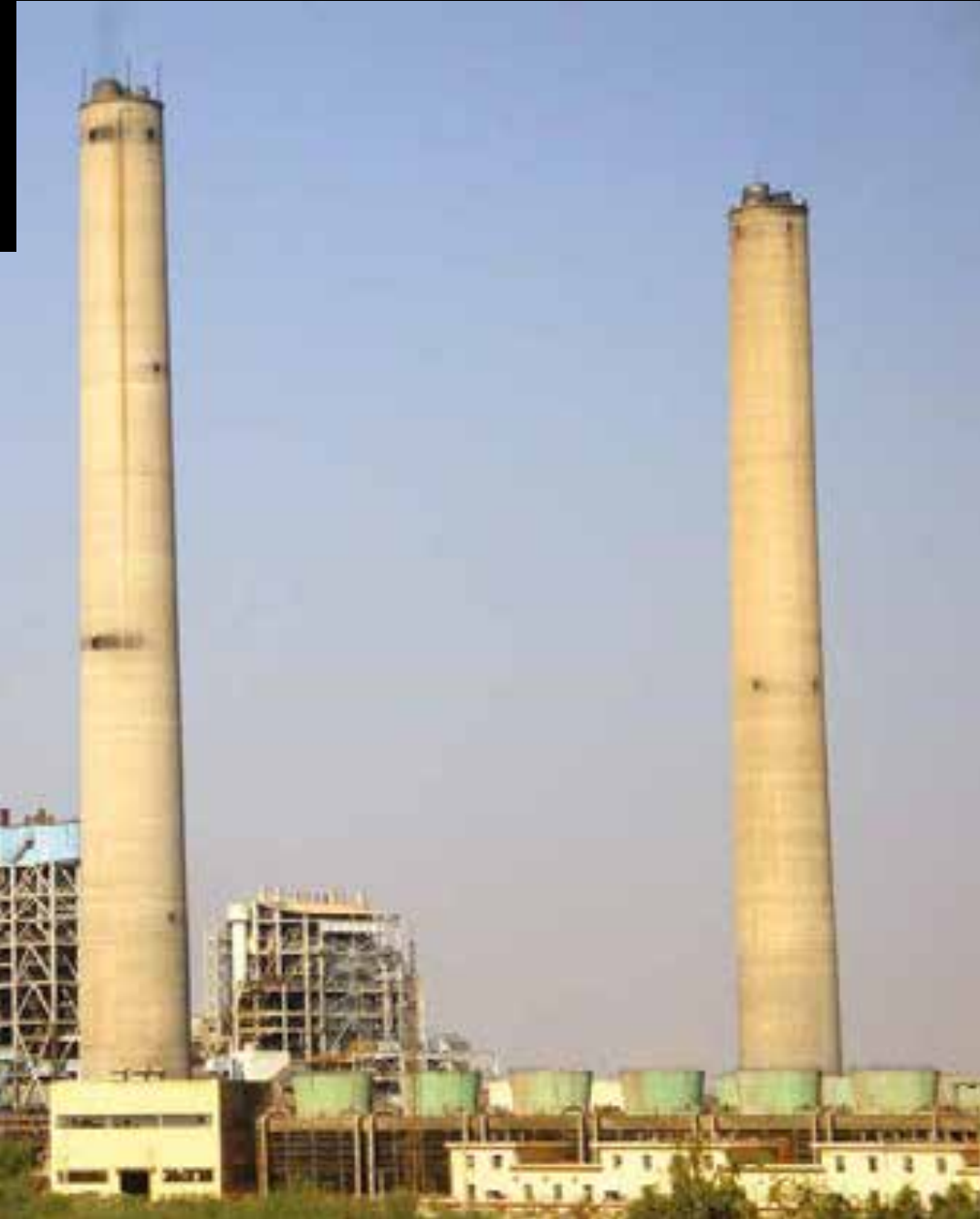
USAID REHABILITATED THE JAMSHORO POWER STATION AND RESTORED ITS GENERATION CAPACITY.
