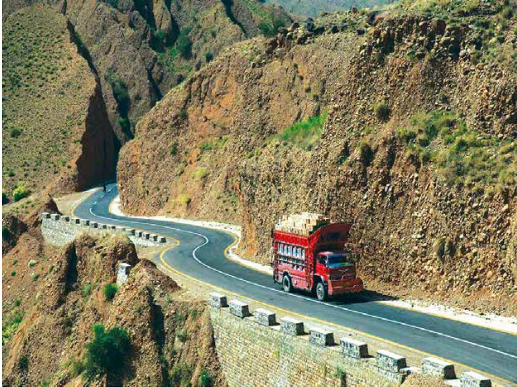
REFURBISHED ROADS REDUCE TRAVEL TIME AND VEHICLE WEAR AND TEAR.
