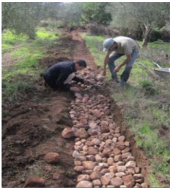
Community members rehabilitate an irrigation system in Figuig. Photo: NEF
